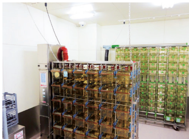
Figure: Two types of Individually Vented Cage systems in new SPF animal facility
